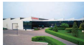
Giacomini S.p.A. Forging plant Castelnovo del Garda (VR) (G3)
